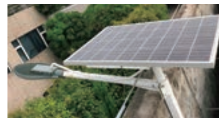
▲ Solar LED-type outdoor lights
